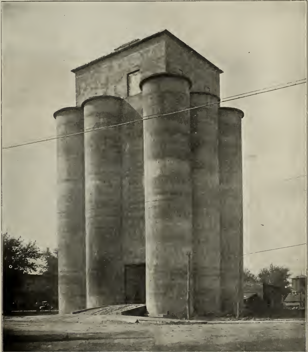
NEW ELEVATOR OF THE MONTELIUS GRAIN COMPANY, PIPER CITY, ILL.
